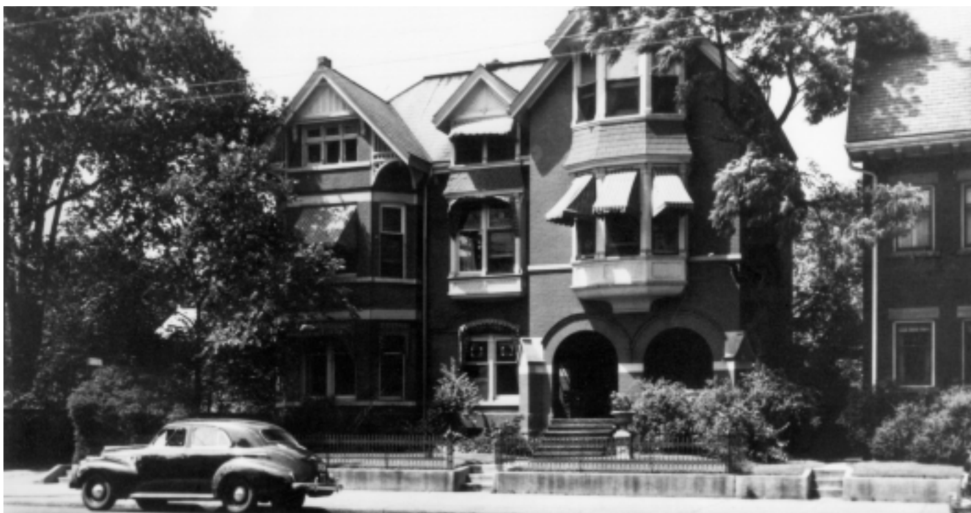
Figure 20 The former Meadonia Hotel served as the first campus of the CMCC, 1945–1969; from the October 1945 issue of the Journal of the National Chiropractic Association .
