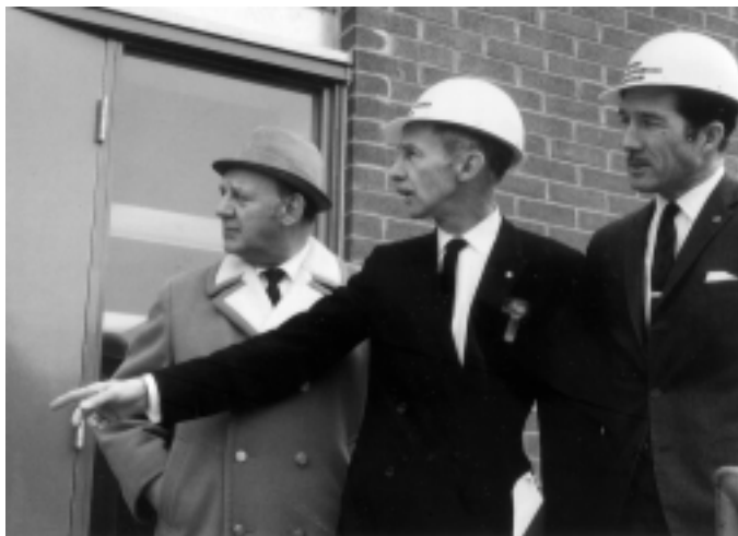
Figure 30 Drs. Howard Gauthier, Earl Homewood and Donald Sutherland inspect progress of CMCC's new campus, 1968.
